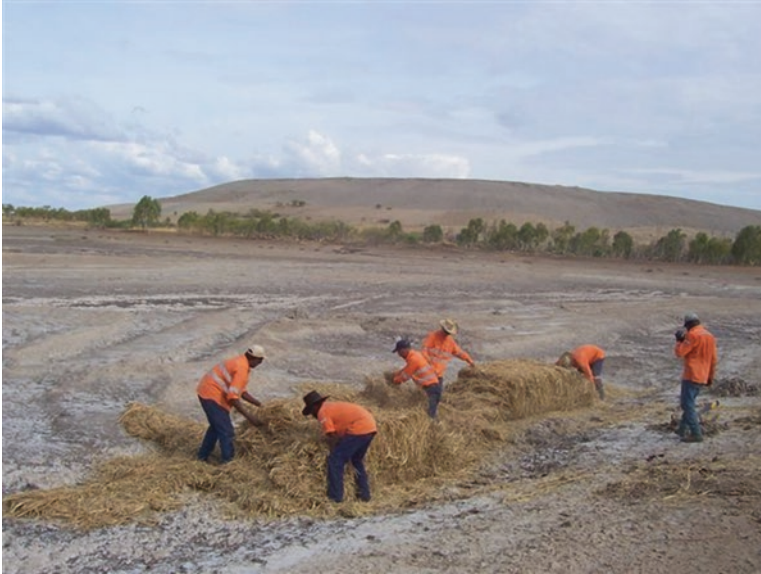
Fig. 6.1 Evaporation pond in northern Queensland, Australia, with straw bales being distributed prior to the monsoon season. (Photograph supplied by Century Mine)
